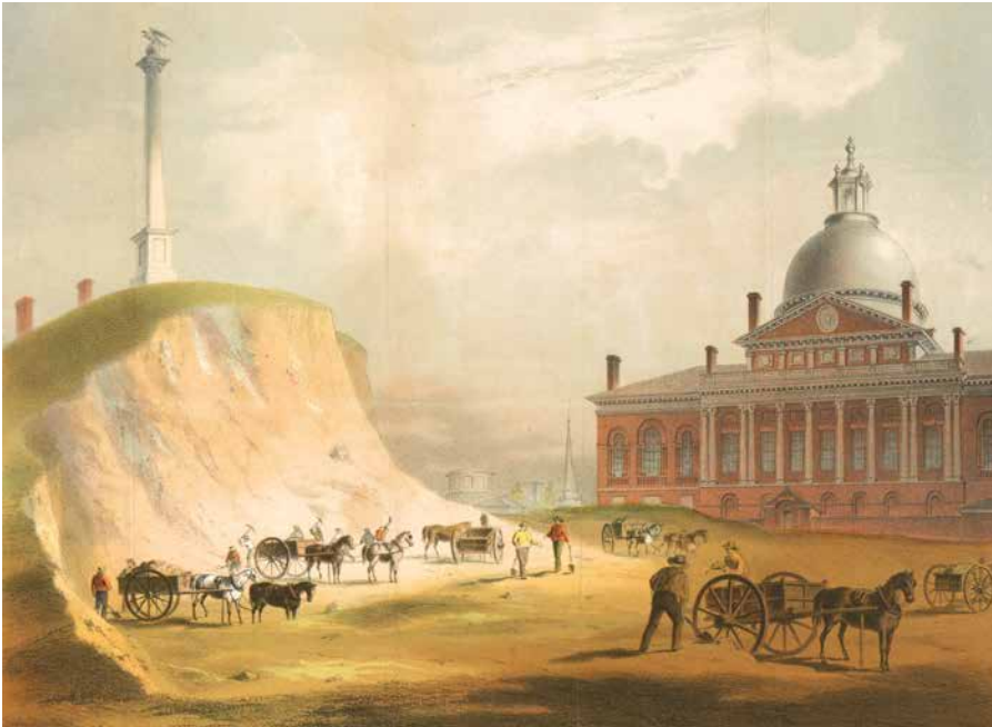
Watercolor by John Rubens Smith, ca. 1810, showing the excavation of Beacon Hill with Charles Bulfinch's State House on the right. Image courtesy Artvee
